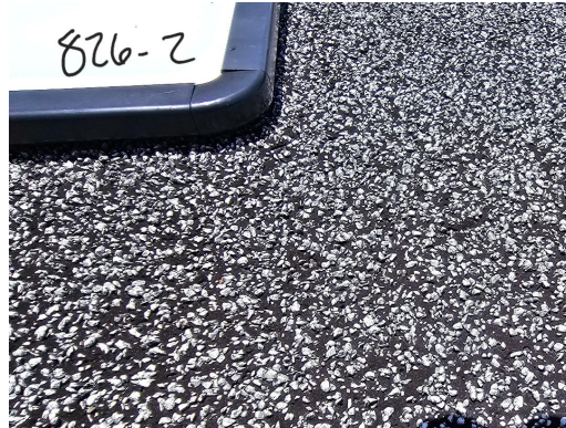
826-2 (Main House) Rolled Asphalt Roofing Typical Exterior Roof
