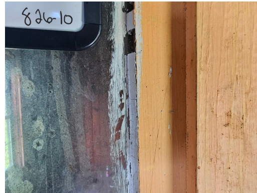
826-10 (Guest House) Glazing/Gray Typical Exterior Windows 2% Chrysotile
