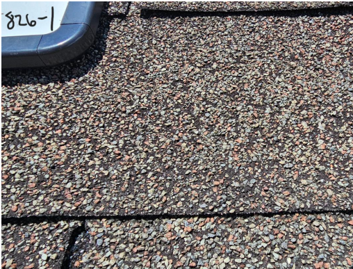
826-1 (Main House) Asphalt Shingle Typical Exterior Roof
