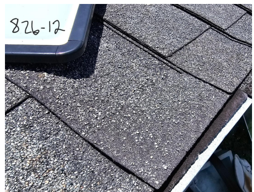
826-12 (Guest House) Asphalt Shingle/Tar Typical Exterior Roof
