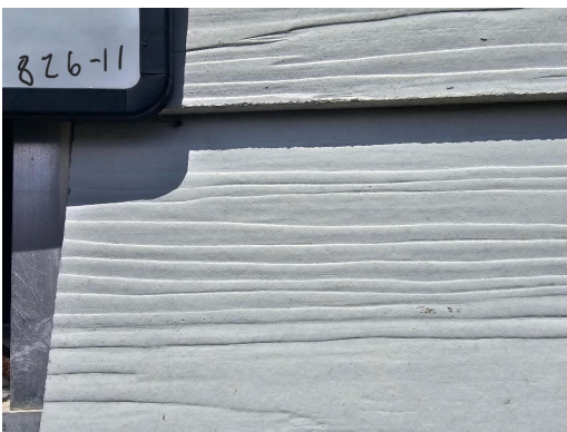
826-11 (Guest House) Siding Typical Exterior Walls
