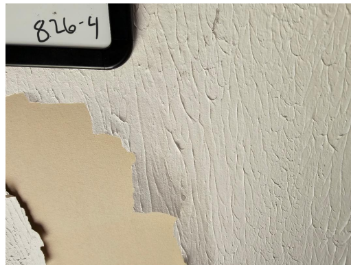
826-4 (Main House) Surfacing Texture Typical Interior Walls/Ceilings
