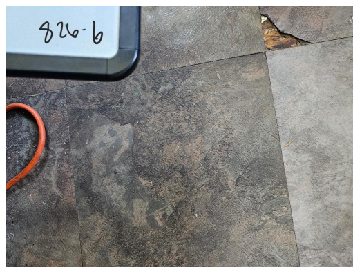
826-6 (Main House) 12"x12" Floor Tile/Adhesive Interior Mud Room
