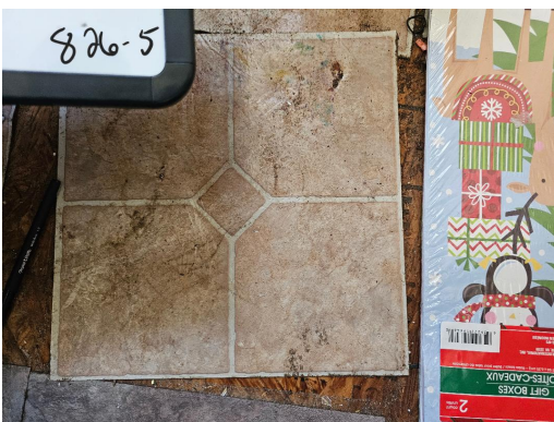
826-5 (Main House) 12"x12" Floor Tile/Adhesive Interior Mud Room
